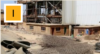
Crown footprint elimination
