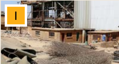
Crown footprint elimination
