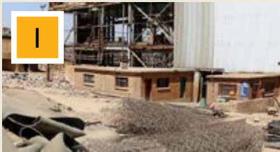
Crown footprint elimination
