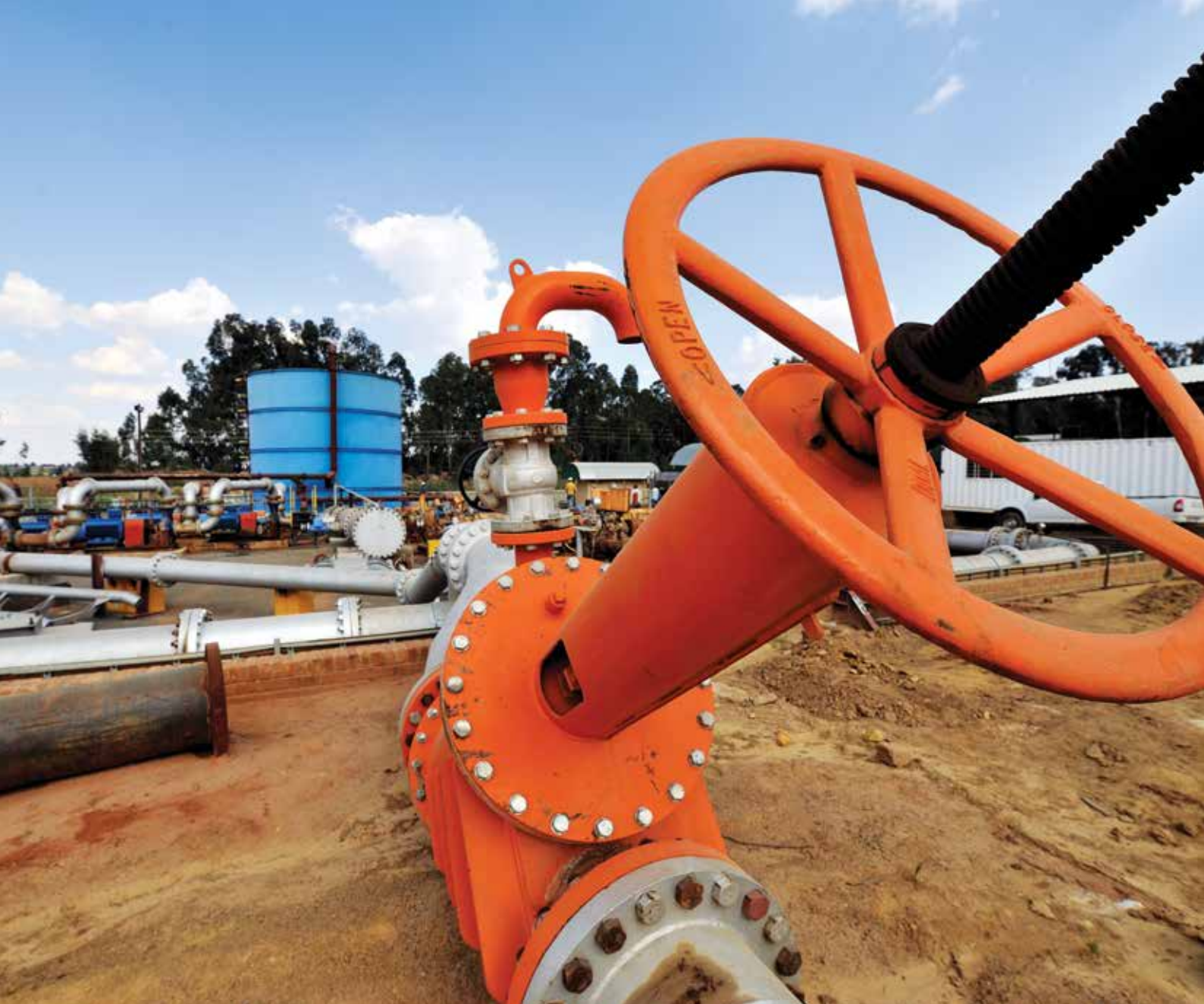
Above: Infrastructure at the Elsburg reclamation site
