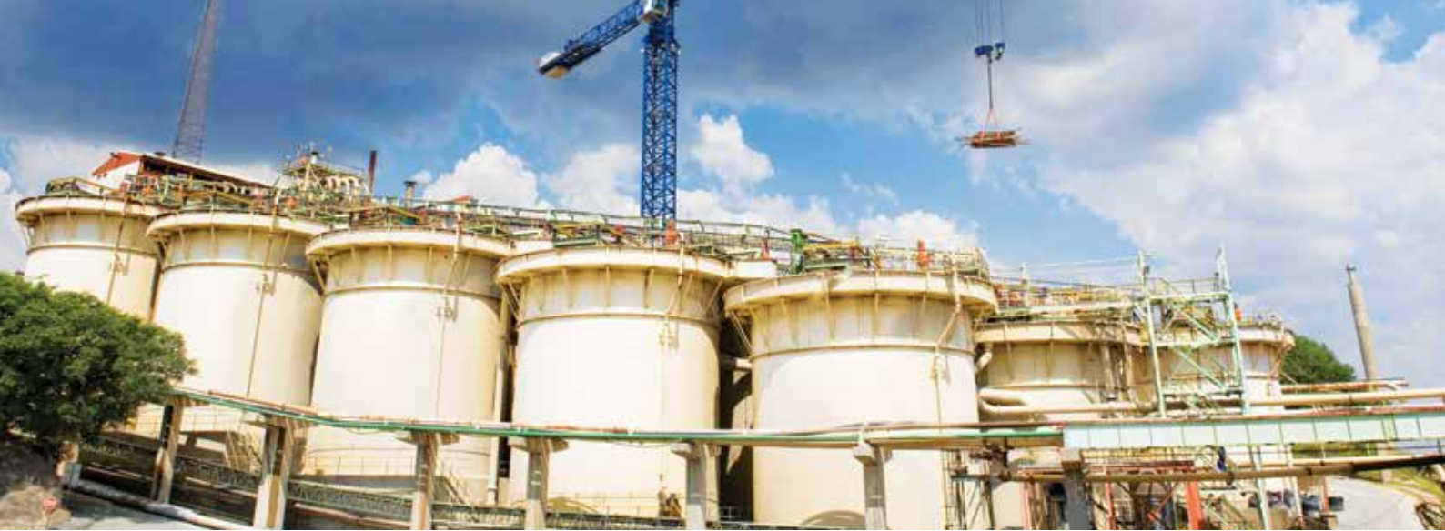
Above: CIL circuit at Ergo's Brakpan plant
