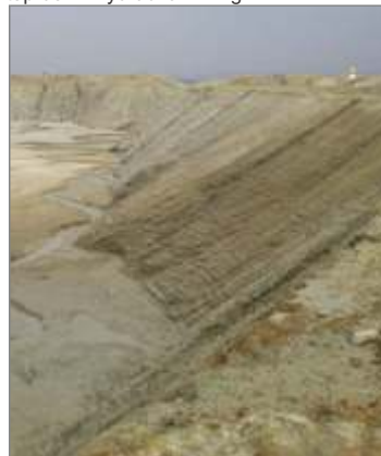
Large consistent slope faces formed by top-down hydraulic mining
